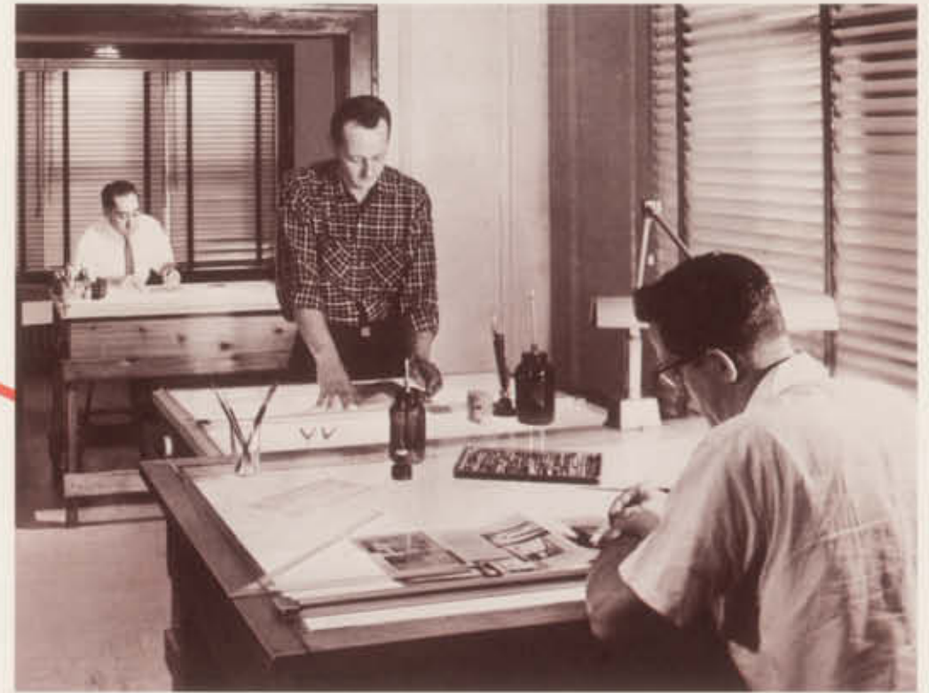
Light tables equipped with parallel arms used for precision assembly.
